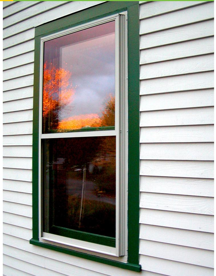
Available as fixed panels or tracked two or three-panel attachments (shown here), exterior modern low-e storm windows are more energy efficient, more durable, and more attractive than older-generation storm windows.
